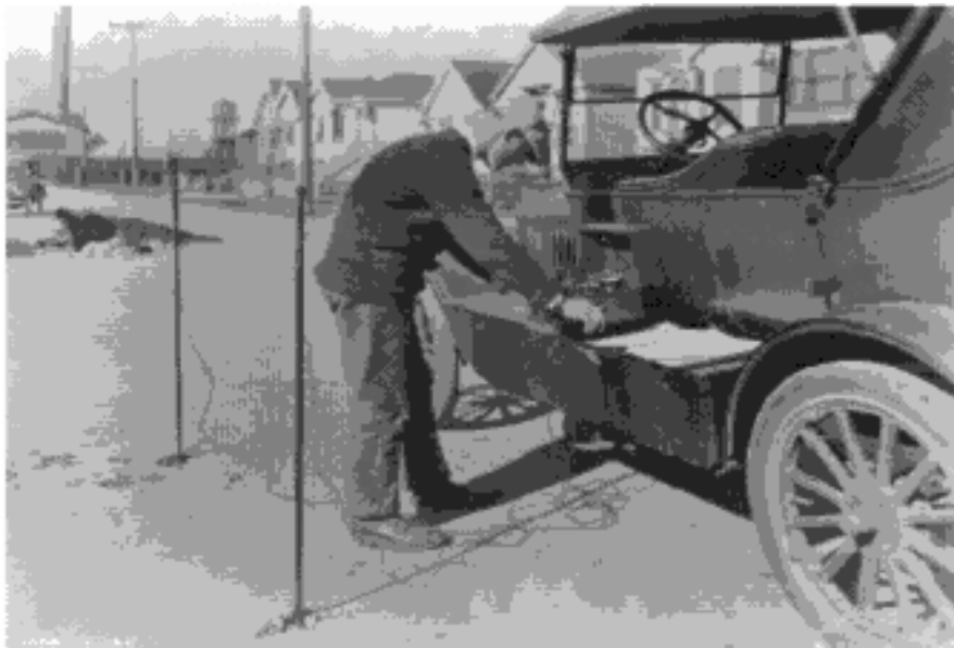
Fig. 11 – Mobile auto-laboratory designed for stray currents monitoring (Los Angeles 1910). In Background (left) it can be observed digging for an underground pipe perforated by stray currents.
