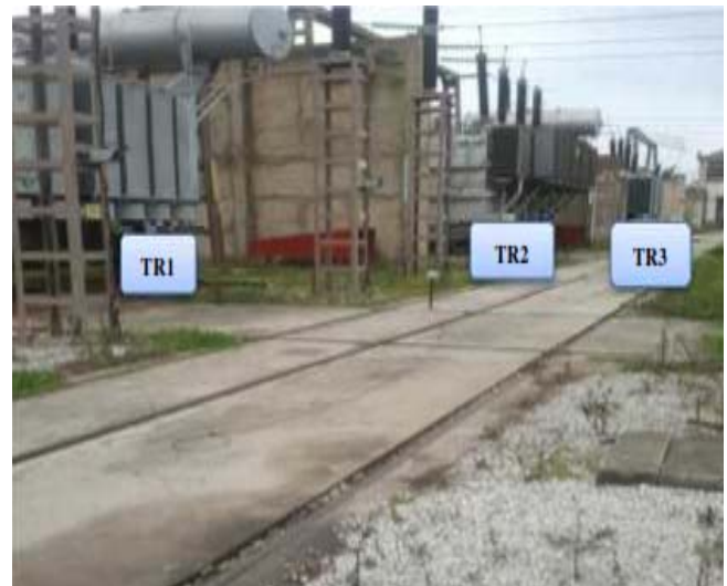
Fig. 3 – Passage of power transformers.
